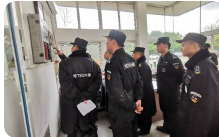
Daily operation training for the fire alarm control panel
