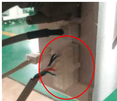
Fig.17 Before the 373D sensor is installed
