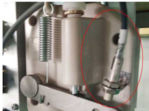
Fig.22 After the sensor is installed
